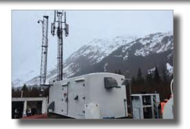
The PowerGen can be optionally outfitted with the Low Temperature Operation Package to extend starting capability and operation down to -40°F (-40°C) for standby systems in cold climates. The Low Temperature Operation Package may not be necessary for continuous-run (prime power) applications in cold climates. Please inquire for more information.
