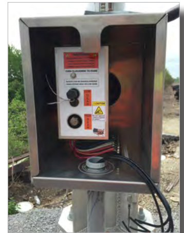
Can be raised and lowered manually (hand-crank) or via a power drill
