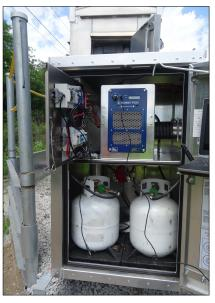
**Fuel Efficient** Consumes <sup>1</sup>/<sub>4</sub> lb LP/hour and can provide 130-160 hours of runtime on two (2) standard BBQ propane tanks.
