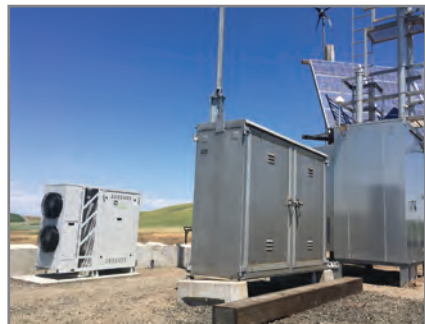
Pilot test site with major class I railroad. PTC location where existing solar & wind system couldn't meet daily demand until the PowerGen was installed in June 2017.
