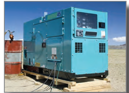
Gas/diesel generators need frequent oil changes (every 25-100 hours) and have an overall design life of 1,000 to 3,000 hours.
