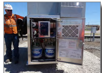
Solid Oxide Fuel Cells are powered by readily available, easily transportable and low cost propane or natural gas.
