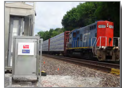
Solid Oxide Fuel Cells have no moving parts, need no oil changes or routine maintenance over their life
