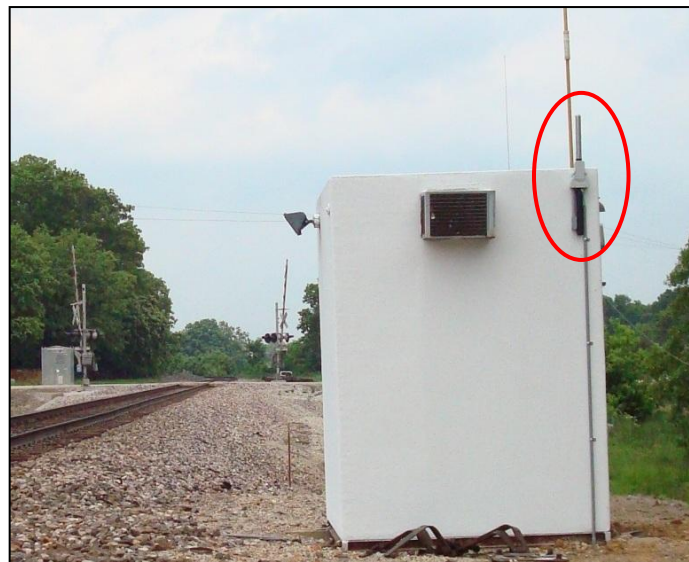
Hot Box Installation
